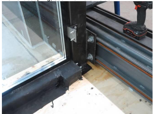
Picture 7 Internal glazing
