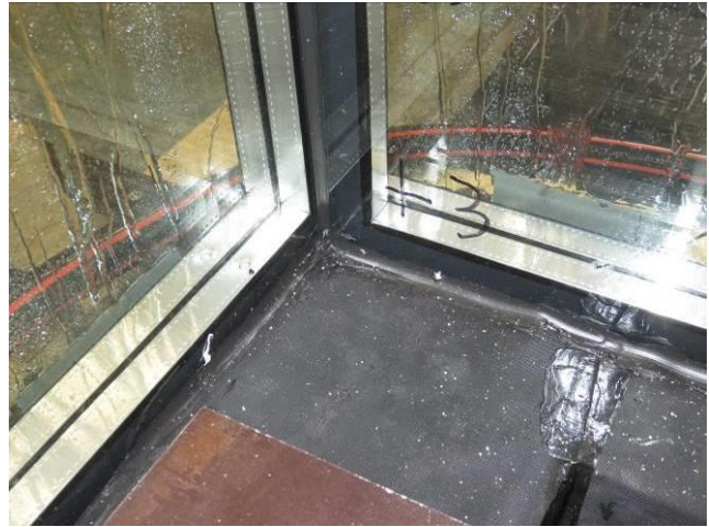
Picture 9 Internal glazing
