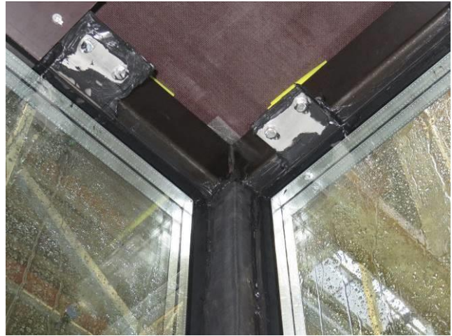
Picture 3 Fixing method of façade construction
