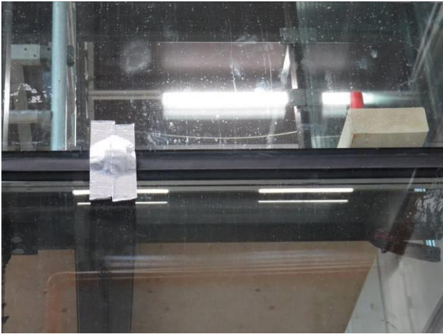
Picture 8 External glazing
