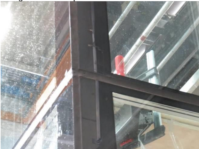
Picture 4 Element coupling, seen from the outside
