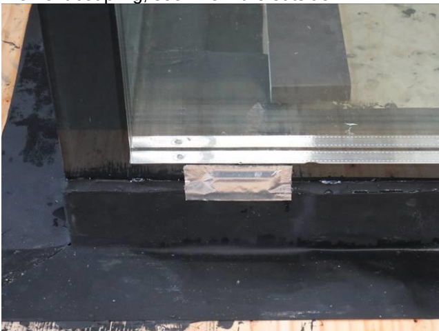
Picture 6 External glazing
