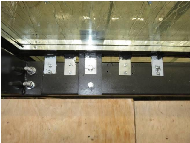
Picture 2 Fixing method of façade construction
